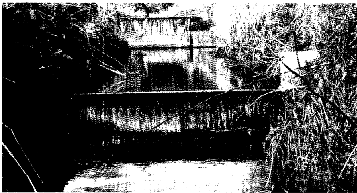
Small weirs allow free passage on the Shiel Burn
