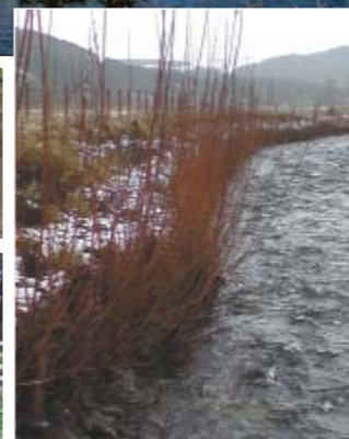
ABOVE: Example of 'soft engineering' in the form of live willow which we hope to protect the banks of the Bogie and Isla
